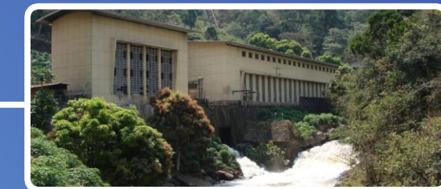
Bendera Hydro Power Scheme ( Future capability of 50MW )
